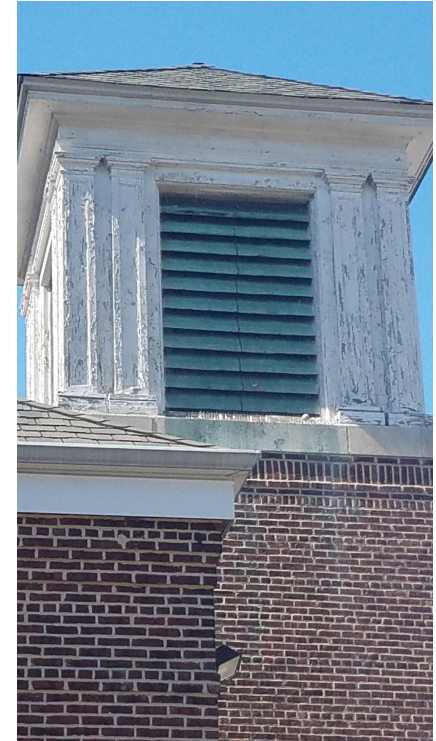
Repaint Main Street School Bell Tower
