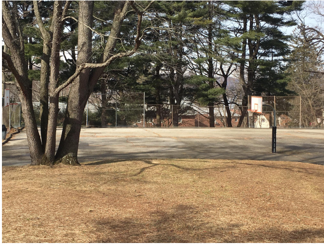
Repave Basketball court
