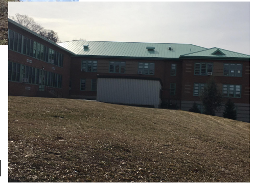
Remove old Storage Shed
