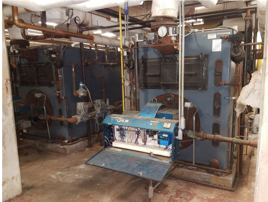
Dows Lane Boiler - Failing pipes and sessions
